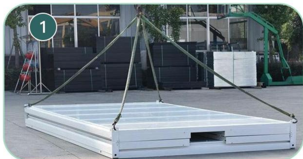
折叠箱房安装清场 (Installation clearance)
